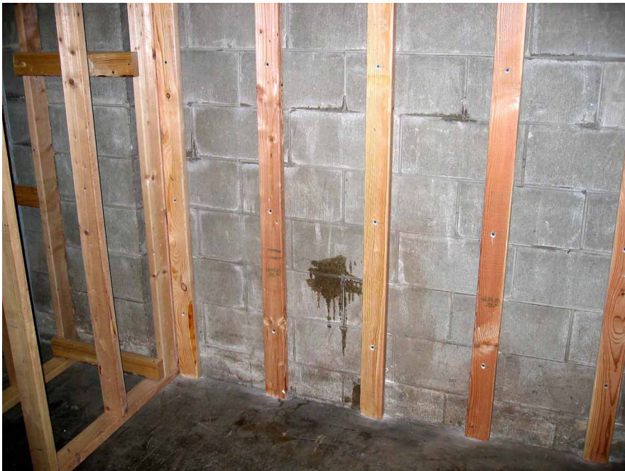
2 x 4 furring strips fastened to concrete block with Tapcon screws.
